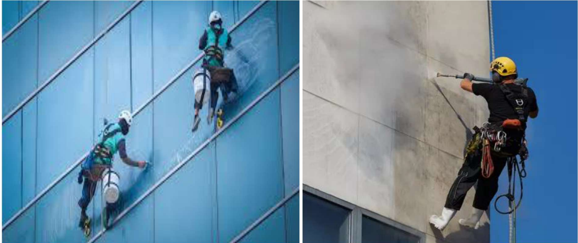
Fig. 1: Window Cleaners And Steam Hose Used In Façade
